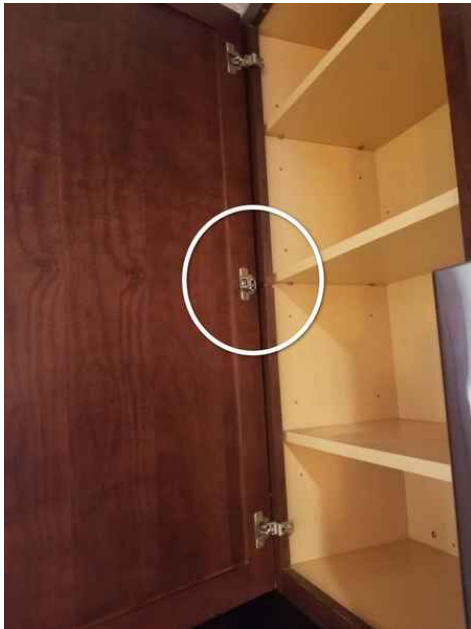
hinge not connected
